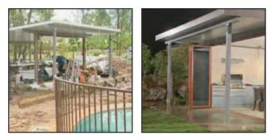
**Deck:** Scottie prepared the area around the pool. 100mm of roadbase was then compacted. Sleepers were used as bearers, directly laid on the ground, using a straight edge to make sure they were all level to each other. 140x45mm merbau hardwood was used as decking boards. These were screwed into position using galvanised bugle head screws.
